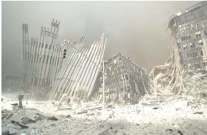
Figure 3-5 - The north wing of WTC4, as viewed from Church Street, looking west, appears surgically removed from the main body of WTC4, which has essentially disappeared. If WTC2 fell on it and squashed the main building, where is the part of WTC2 that did this?
