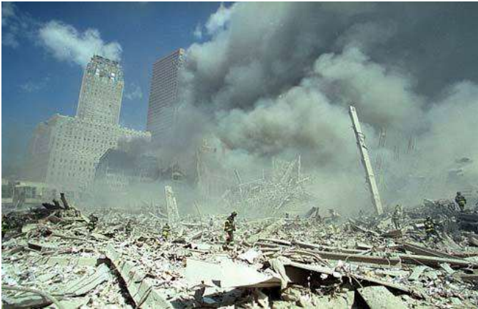
Figure 164 - WTC site immediately after destruction of WTC 1 and 2
