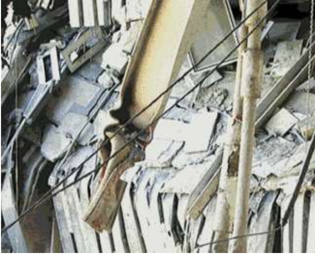
Figure 171 – Inside Banker’s Trust/Deutsche Bank building after WTC destruction.
