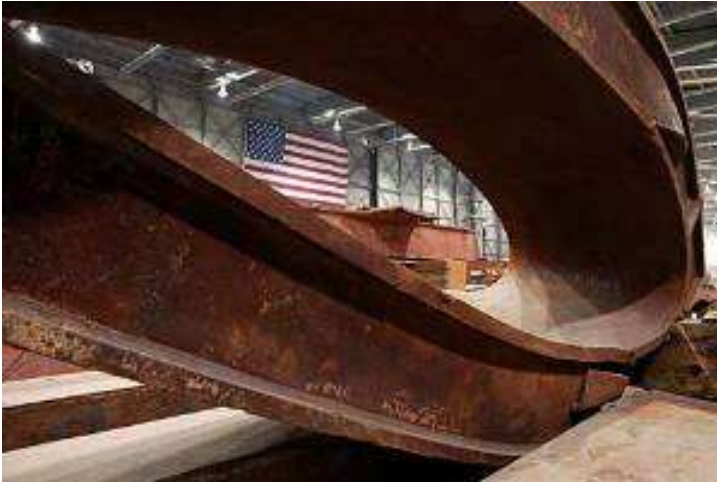
Figure 166 - WTC beam - deformed.
