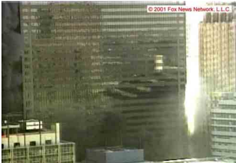
Figure 5–157. Frame taken from a video clip shot from the northeast, showing the north face of WTC 7 within a few minutes of the WTC 7 collapse at 5:20:52 p.m. The intensity levels were adjusted.
