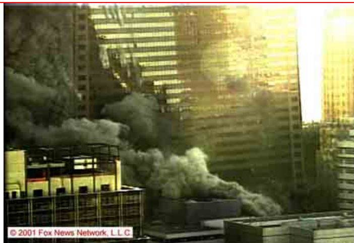
Figure 5–209. Frame from the Camera 6 video clip in Figure 5–189, showing the north face of WTC 7 10.0 s \pm 0.2 s after the east penthouse began to descend. The intensities have been adjusted.
