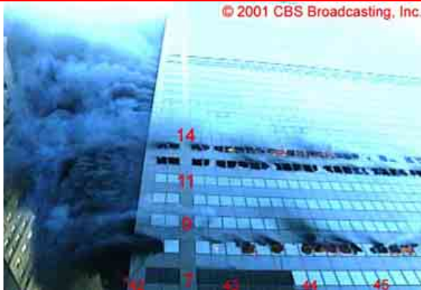
Figure 5–141. Frame from a video shot from near the corner of West Broadway and Barclay Street showing the eastern side of the north face of WTC 7 between 3:53 p.m. and 4:02 p.m. The intensities have been adjusted, and column and floor numbers have been added.
