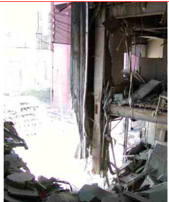
Figure 2–31. Interior view of damage to the north face of 130 Liberty Street by debris falling from WTC 2.
