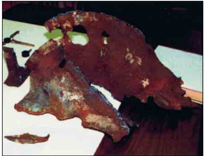
Figure 75. This piece of steel thought to be from WTC7 appears partially disintegrated. (Figure C-1. Eroded A36 wide-flange beam.) (2002) Source: http://www.fema.gov/pdf/library/fema403_apc.pdf
