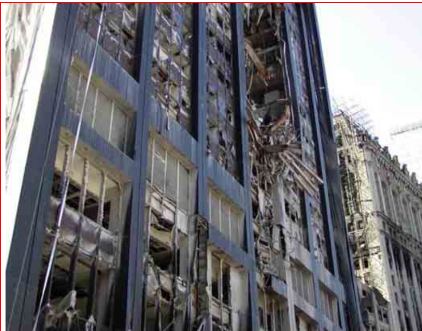
Figure 2–30. Exterior view of damage to the north face of 130 Liberty Street by debris falling from WTC 2.
