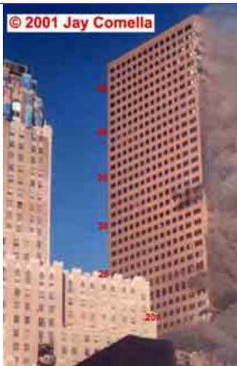
Figure 5–24. Cropped photograph of the west face of WTC 7 shot from West Street between 3:30 p.m. and 4:30 p.m. on September 11. The structure on the left is the Verizon Building, and the building just visible at the bottom is WTC 6. The intensity levels have been adjusted.
