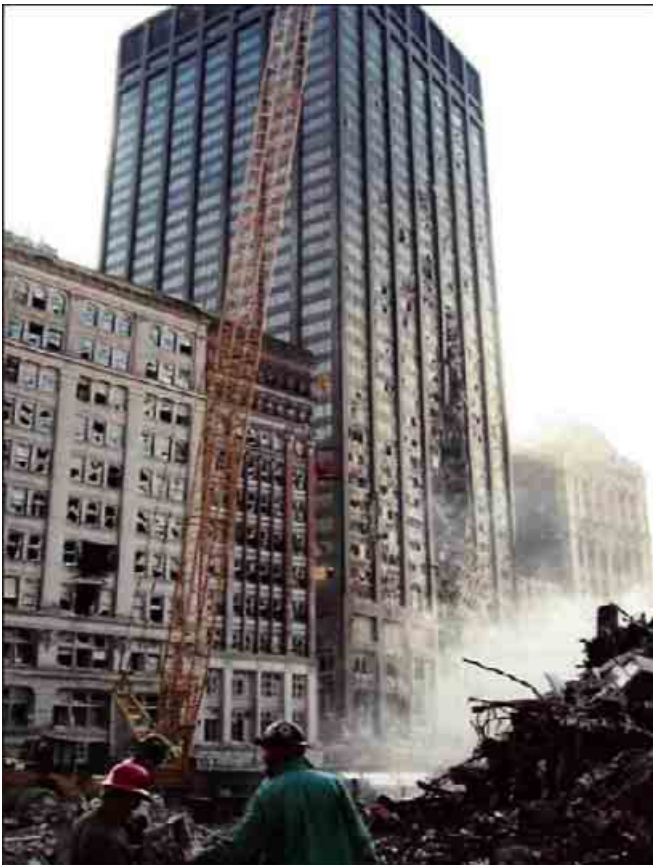
Figure 6-1 North face of Bankers Trust building with Impact damage between floors 8 and 23.
