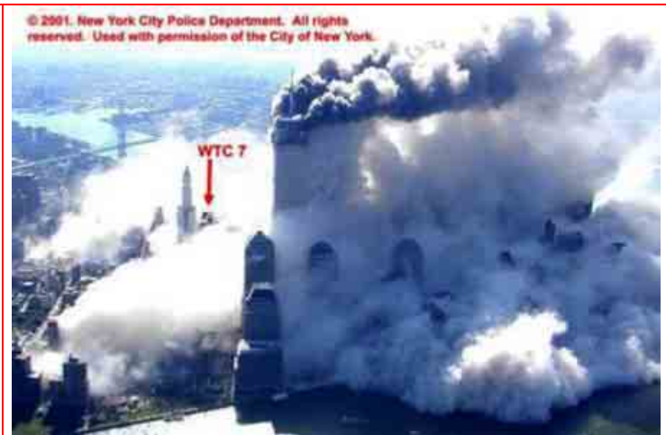
Figure 5–27. Cropped photograph showing the dust cloud created by the collapse of WTC 2. The image was shot from the west at 10:03:56 a.m. WTC 7 can barely be seen above the cloud. The intensity levels of the photograph have been adjusted.
