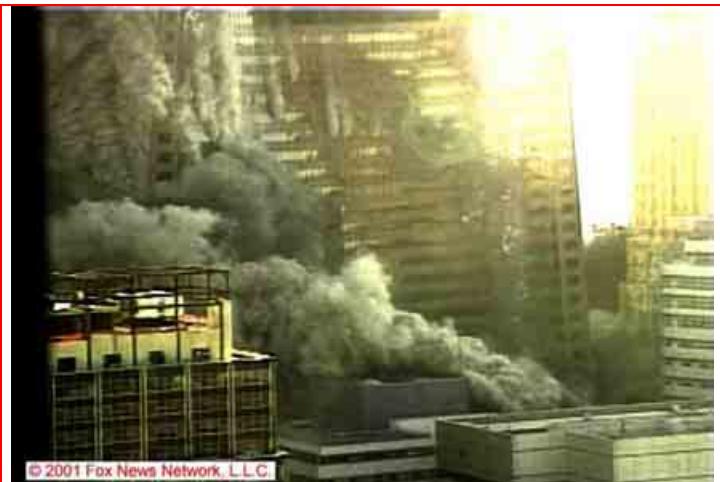
Figure 5–212. Frame from the Camera 6 video clip in Figure 5–189, showing the north face of WTC 7 11.0 s \pm 0.2 s after the east penthouse began to move downward. The intensities have been adjusted.
