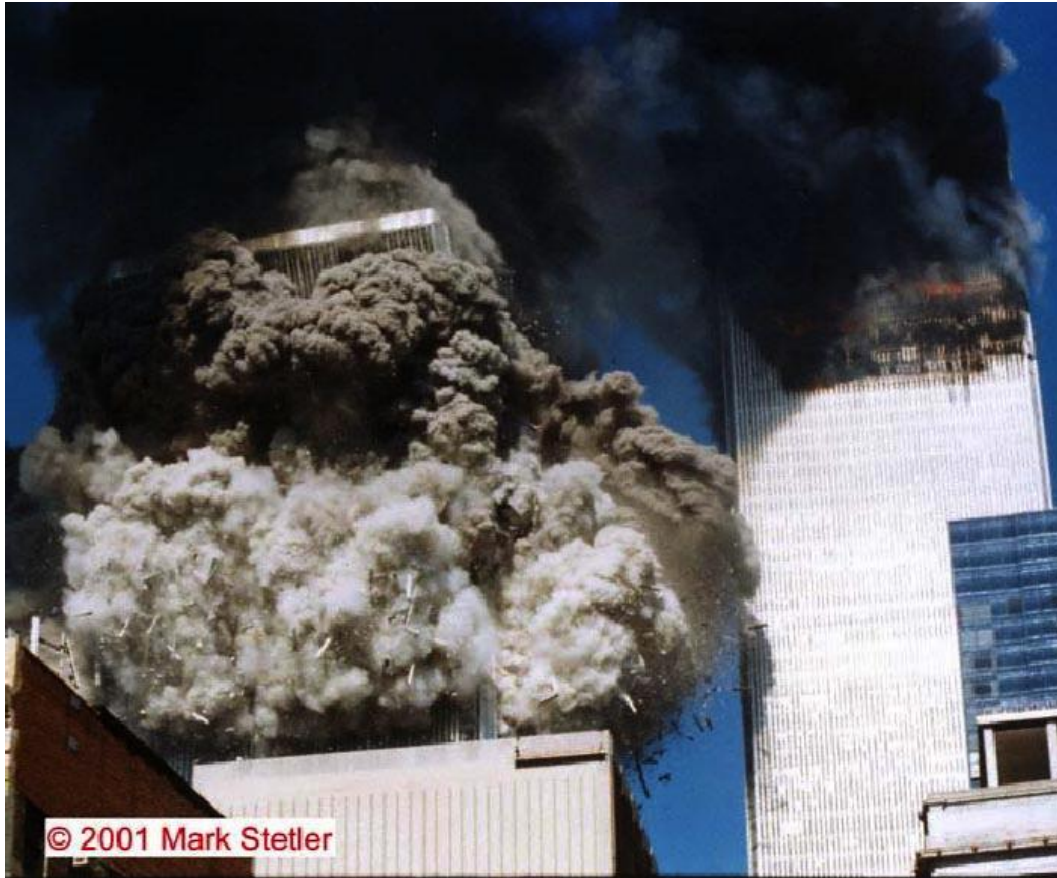
Figure 3-5. Photograph of WTC 2 tilting to the southeast at the onset of collapse.
