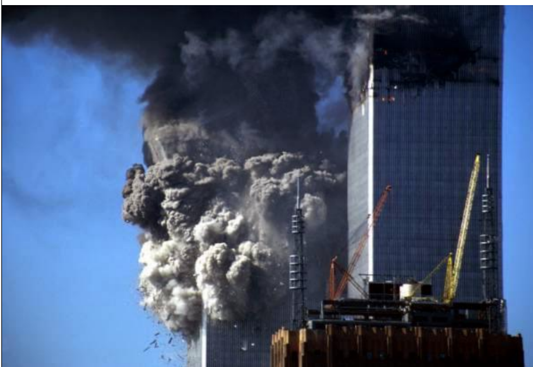
Figure 13. WTC2 tipping eastward, as viewed from the north. The tipping top is disappearing
