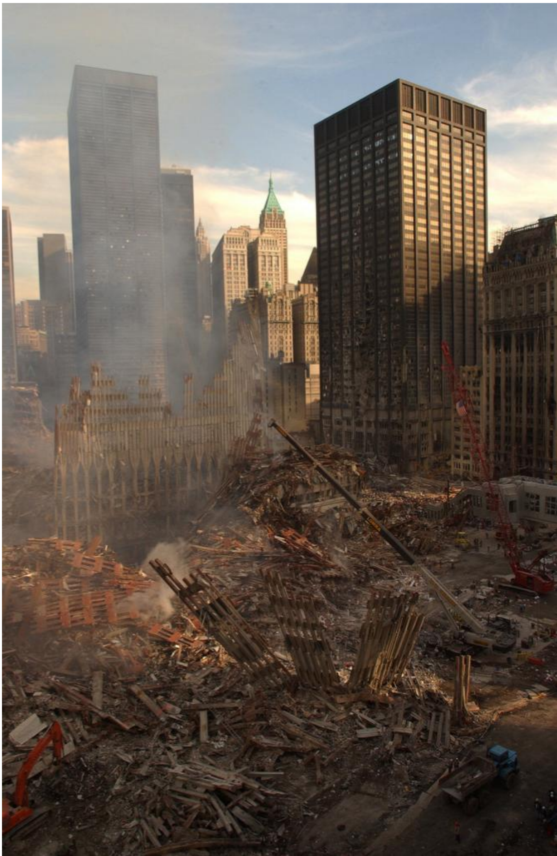
Figure 19. The three steel wheatchex stabbed into West Street in the foreground and the remains of WTC3 in the background, in front of the west wall of WTC2.
