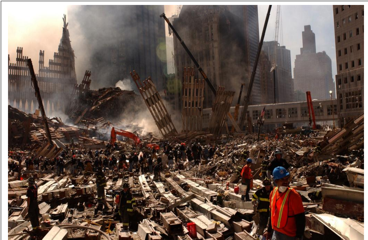
Figure 20. The remarkable "lay down" of steel wheightex from the lower stories of WTC1 on West Street (West Side Highway). The WTC3 debris pile is in the background, next to the unsupported WTC2 wall. (9/13/01)
