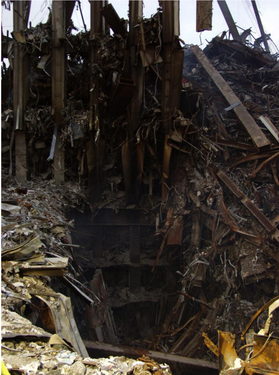
Figure 18. This hole adjacent to WTC2 (zone 2 in Figure 303(c)) is through sidewalk and pavement. This hole contains more debris than the hole discussed in Figure 300 above. It looks as if the debris fell in the hole. Note the scale, shown above. (photo filed 9/21/01)
